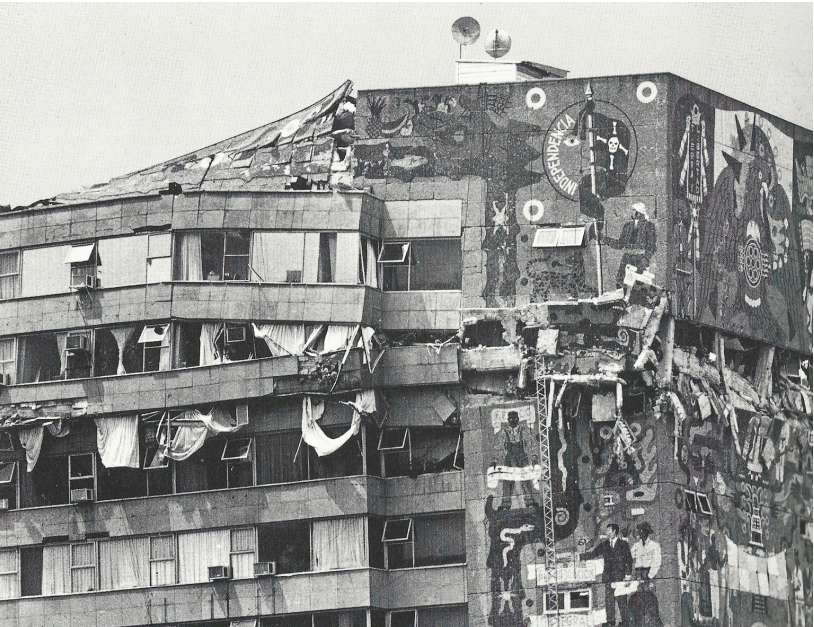
Fig. 01 Centro SCOP (c. 1954). Damaged portion of the building after the 1985 earthquake. The building was then lowered from ten floors to seven. In 2017, another massive earthquake (magnitude 7.1) struck central Mexico.
